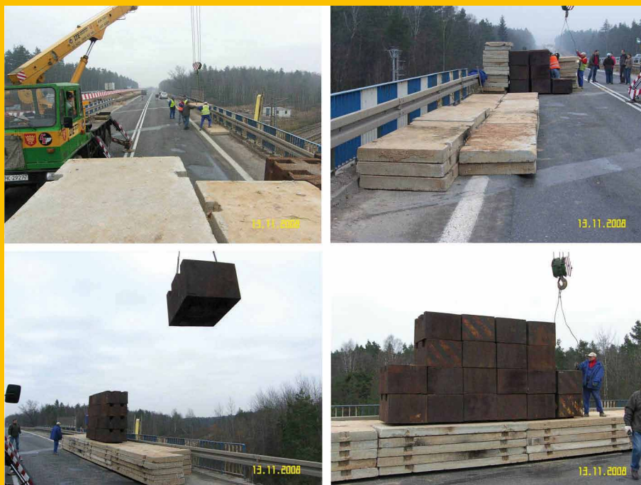
Figure 2.4 Proof load testing execution on the bridge
