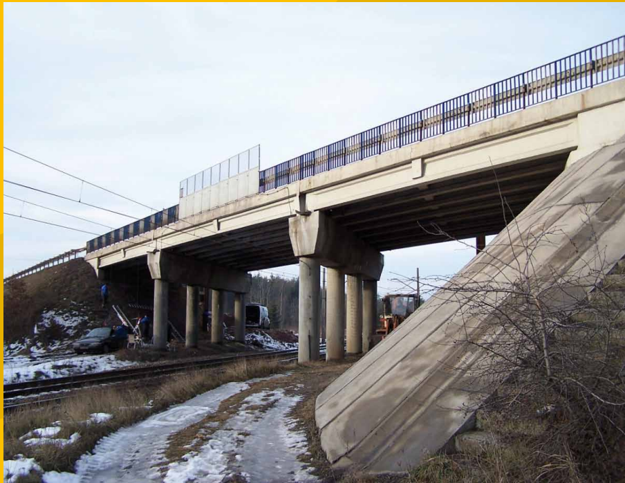
Figure 2.3 General view of the Barcza bridge
