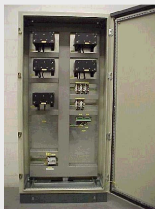
Montage LIDA35 Titanium anodesysteem
