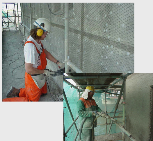
Montage LIDA35 Titanium anodesysteem
