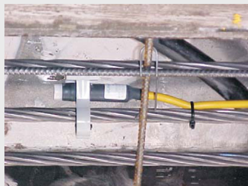
ERE-20 elektrode in damwand
